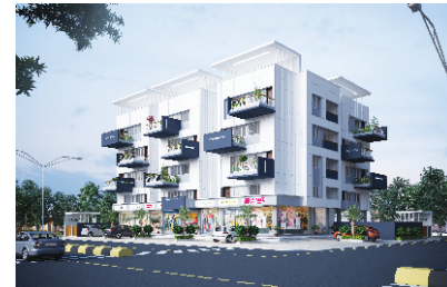
Creative Homes AURAA Katol Main Road, Nagpur
